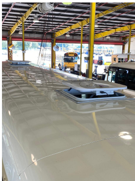
Picture 3 Both Roof Hatches Opened
